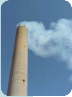
Coleson Cove Generating Station
