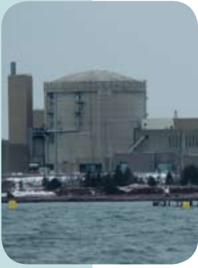
Point Lepreau Nuclear Station
