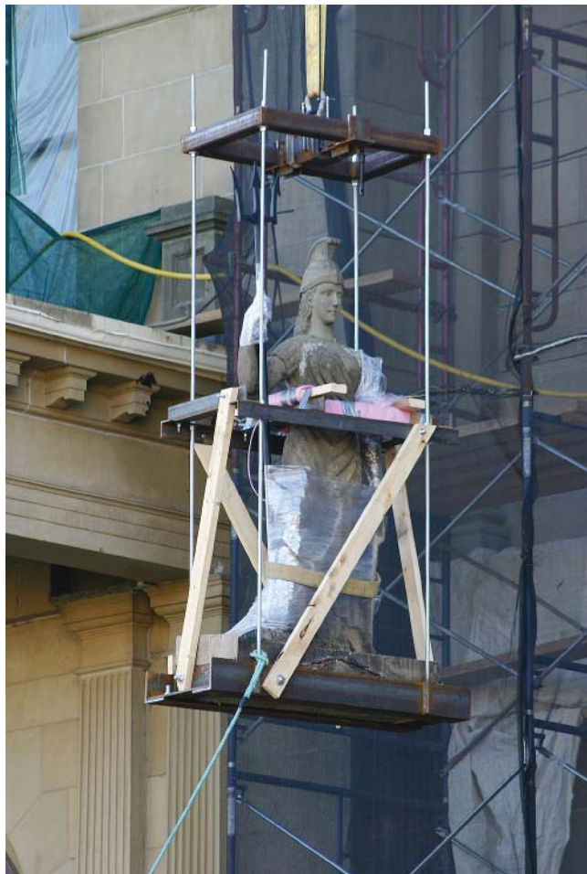
The sculpture Britannia being lowered. Height: about 2.4 metres (8 feet), width: about 0.9 metres (3 feet) and weight: estimated at over 1500 kg (3,300 lbs).
